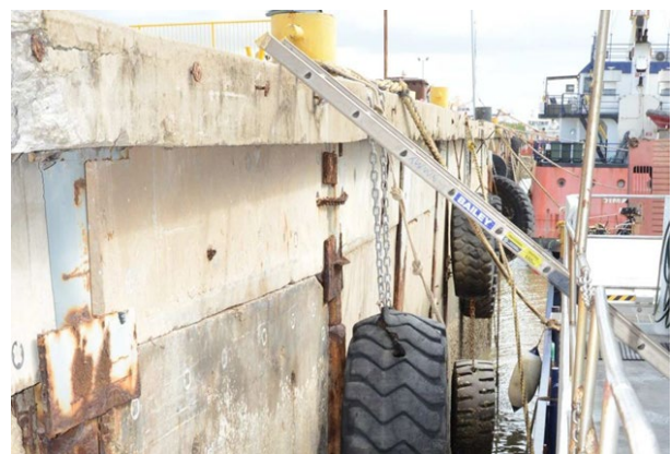
Example of unacceptable access to a vessel, the unsafe conditions amplified at low tide
